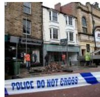
Chimney collapses onto Durham's North Road
